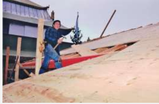
Building roof of East Wing
